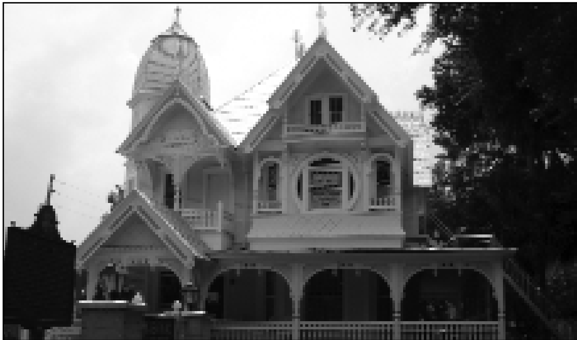
The Donnelly House, a Mount Dora landmark since 1893, is a prime example of the beautiful, varied architectural styles found throughout the city.
